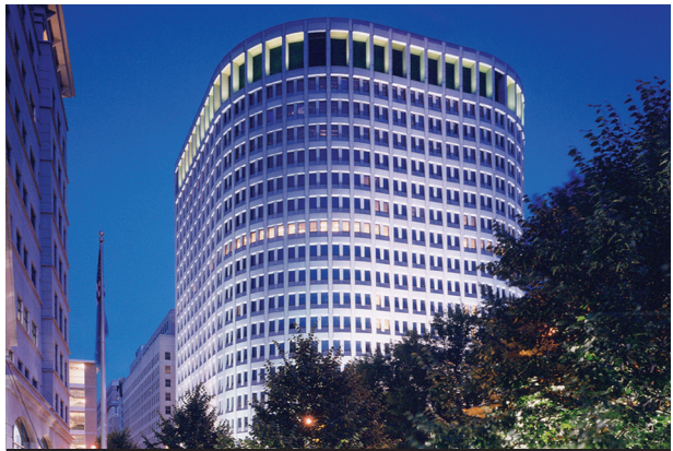
The Brandywine Building
